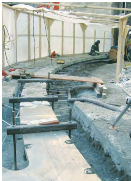
New carriage track for sector gates at the Iroquois Lock
