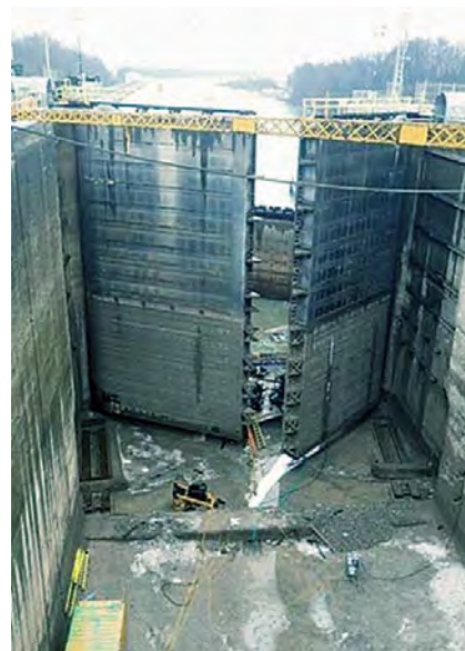
Lock 1 – Heel cast girder replacement for gates 1 and 2
