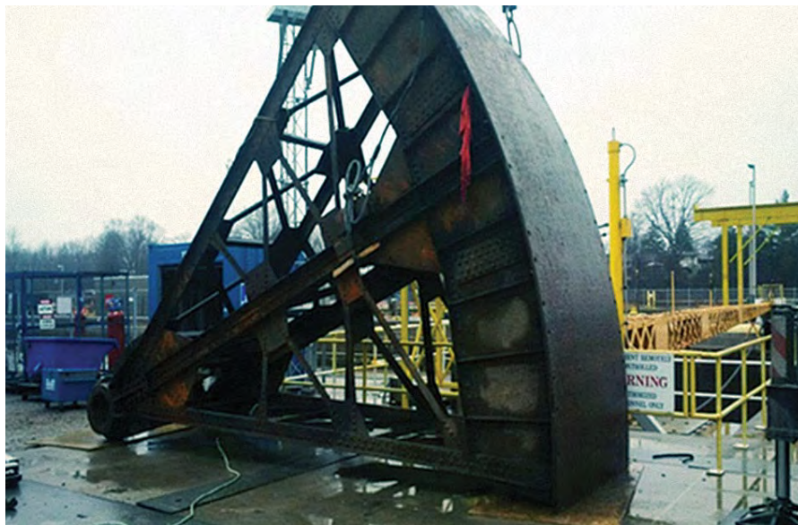
Lock 5 and 6 – Recoating and rehabilitation of side seals and trunnions for valves 1 and 2
