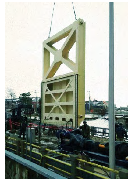
Weir 2: Rehabilitation and replacement of valves and drive machinery
