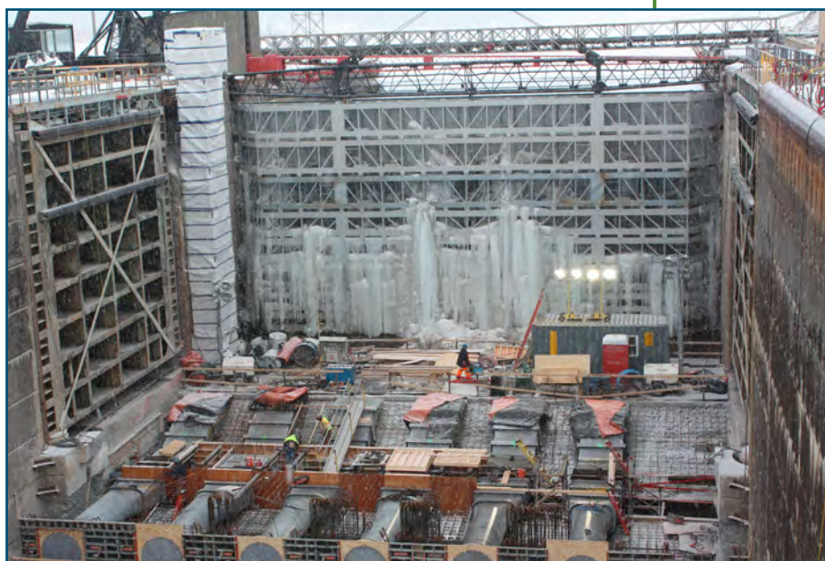
Installation of the new ice flushing system at Snell Lock, Massena, New York.
