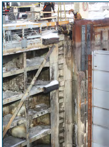
Contractor is working on the downstream north miter gate leaf at Eisenhower Lock.
