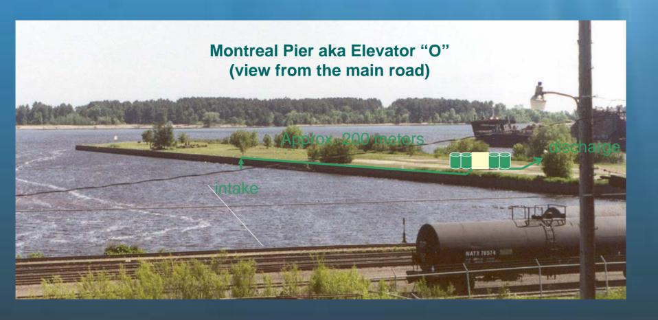
Four 200 cu m tanks; 340 cu m per hr flow; Can recirculate from tanks to treatment to tanks; On site sample analysis and nearby university labs
