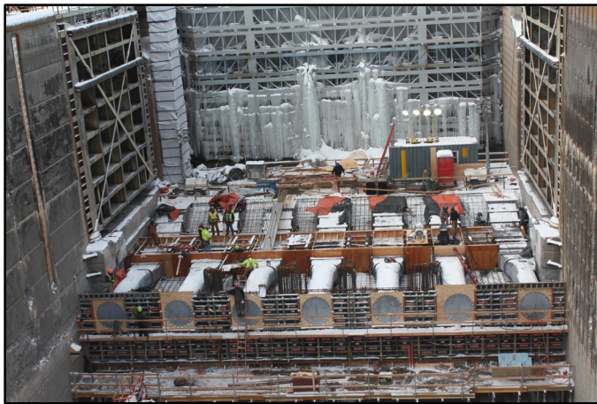
View of the new ice flushing system installation in the Snell Lock chamber in February 2013.
