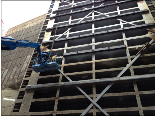
Contractors work on the north downstream miter gate diagonals at Eisenhower Lock.
