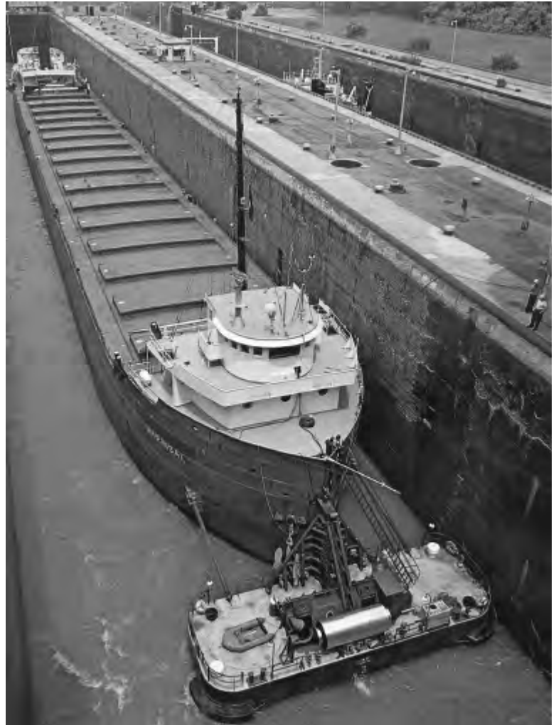
The Seaway purchased two old vessels to test the shunters on the water. This photograph shows a particularly successful test of the Marinsal on the Welland Canal, circa 1979.
