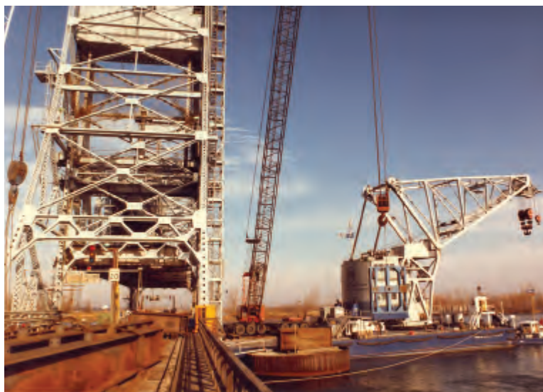
The Seaway Authority had to bring a self-propelled barge, equipped with a 250-foot boom, up from Montreal to remove the damaged shaft and sheave. This photo depicts the barge and the platform of the bridge where it stopped, one-quarter of the way up. ST. LAWRENCE SEAWAY MANAGEMENT CORP.
