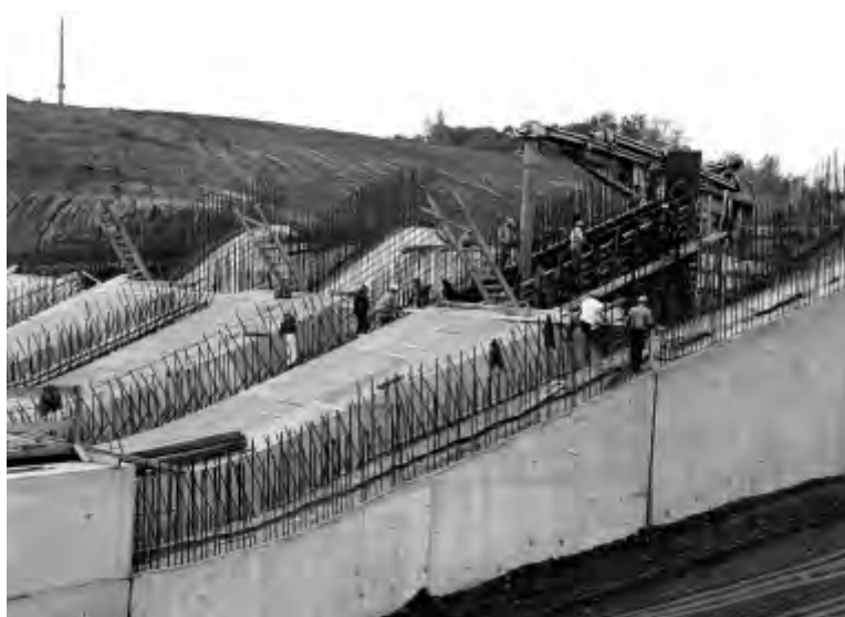
The Main Street tunnel, top, under construction in the summer of 1971. All rail and road traffic would go under the new channel to ensure safer, more efficient navigation. Below, siphon culverts were constructed to handle the flow of the Welland River. ST. LAWRENCE SEAWAY MANAGEMENT CORP.
