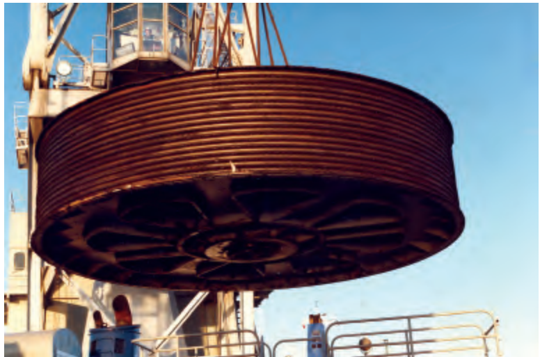
A crane lowers a sheave, fifteen feet in diameter, from the tower of the Valleyfield Bridge. These giant pulleys rotate on a steel shaft and support the sixteen steel cables used to raise and lower the platform of the bridge. Cracks in the shaft prevented the sheave from rotating while the platform was being raised to allow a ship to pass. ST. LAWRENCE SEAWAY MANAGEMENT CORP.
