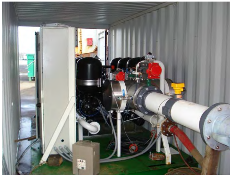
Figure 5 - Hyde Guardian System As Used for Emergency Treatment of Ship Lift Barge "Lucky Angel" in Puget Sound (Hyde Marine, 2009)
