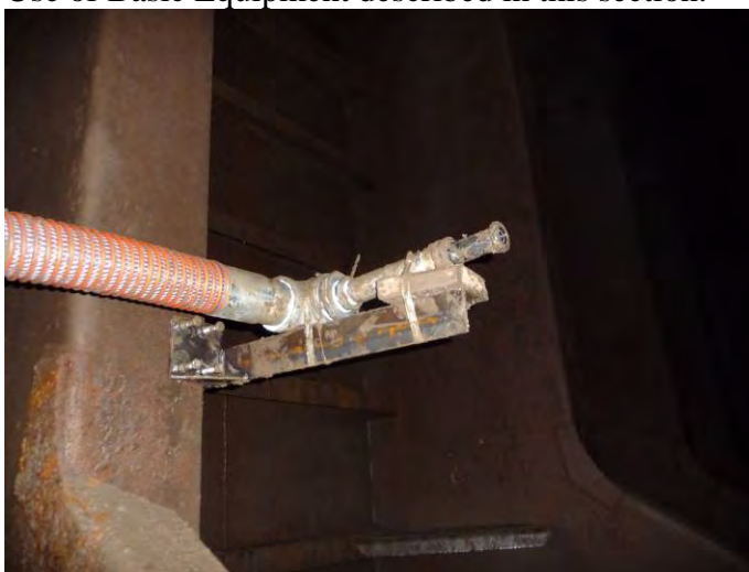
Figure 11 – Nozzle mounted to ship's structure in tank in parallel nozzle arrangement
