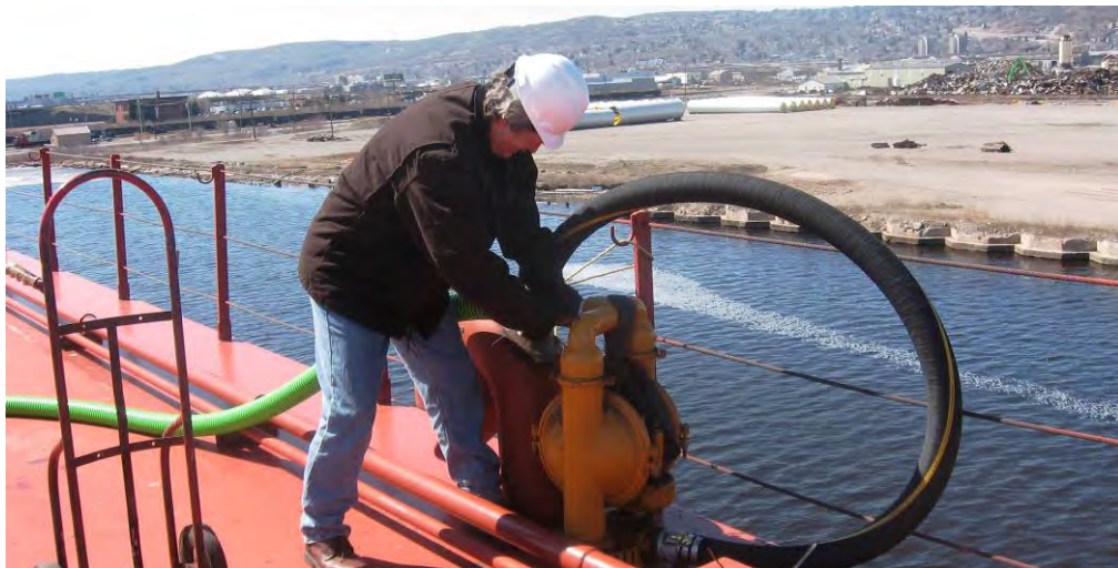
Figure 9 - Rigging Transfer Pump and Hose on Main Deck
